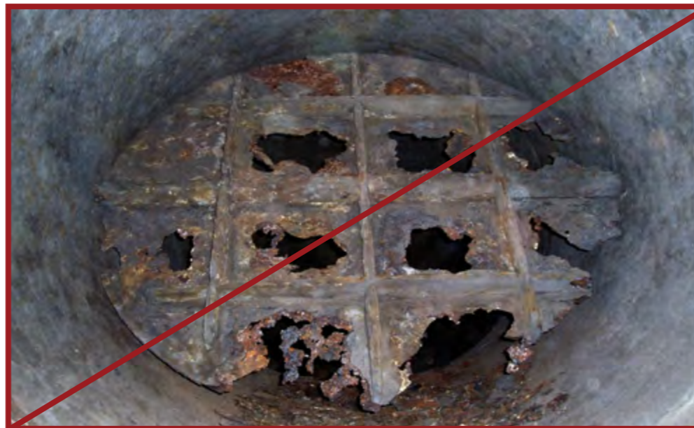
Fire damper that will not pass inspection
