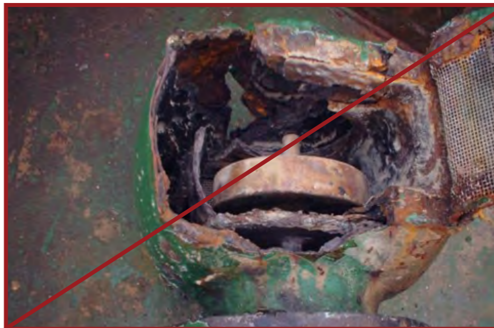
Vent head that will not pass inspection
