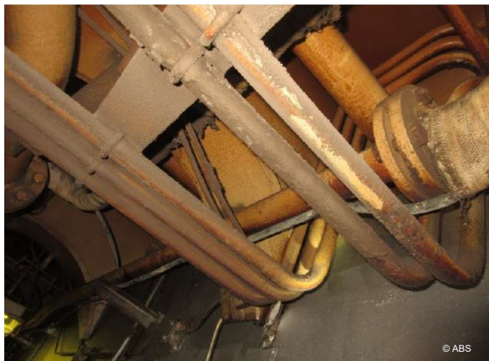
Fuel oil piping and steam piping lacking required insulation
