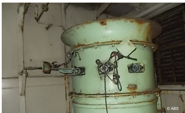
Fire damper linkage defective
