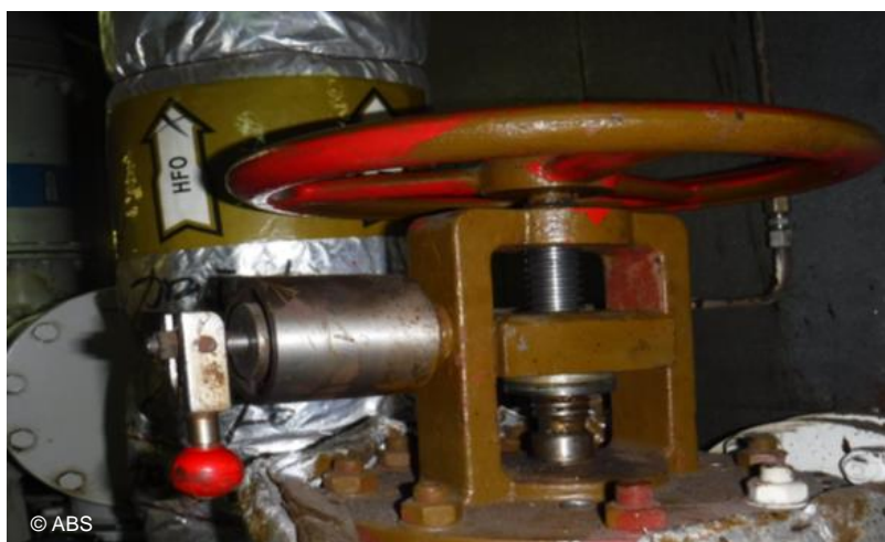
HFO quick closing valve not operable
