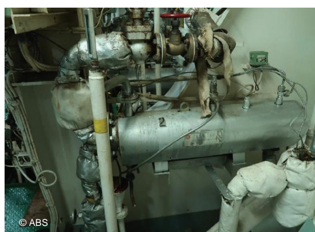
Missing insulation on heaters creates fire hazards
