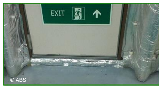
A-60 insulation reinstated
