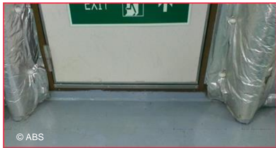
Missing A-60 insulation
